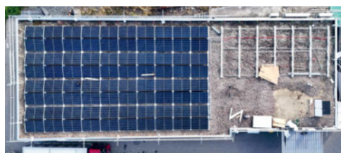
Installation PV-Anlage VOLG, Weier i.E.
