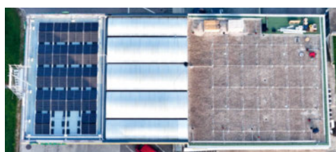
Installation PV-Anlage Dach Tankstelle & AGROLA TopShop Kleindietwil
