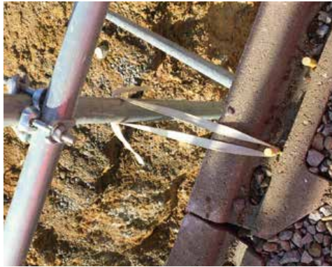
Simple installation of temporary safety railings
