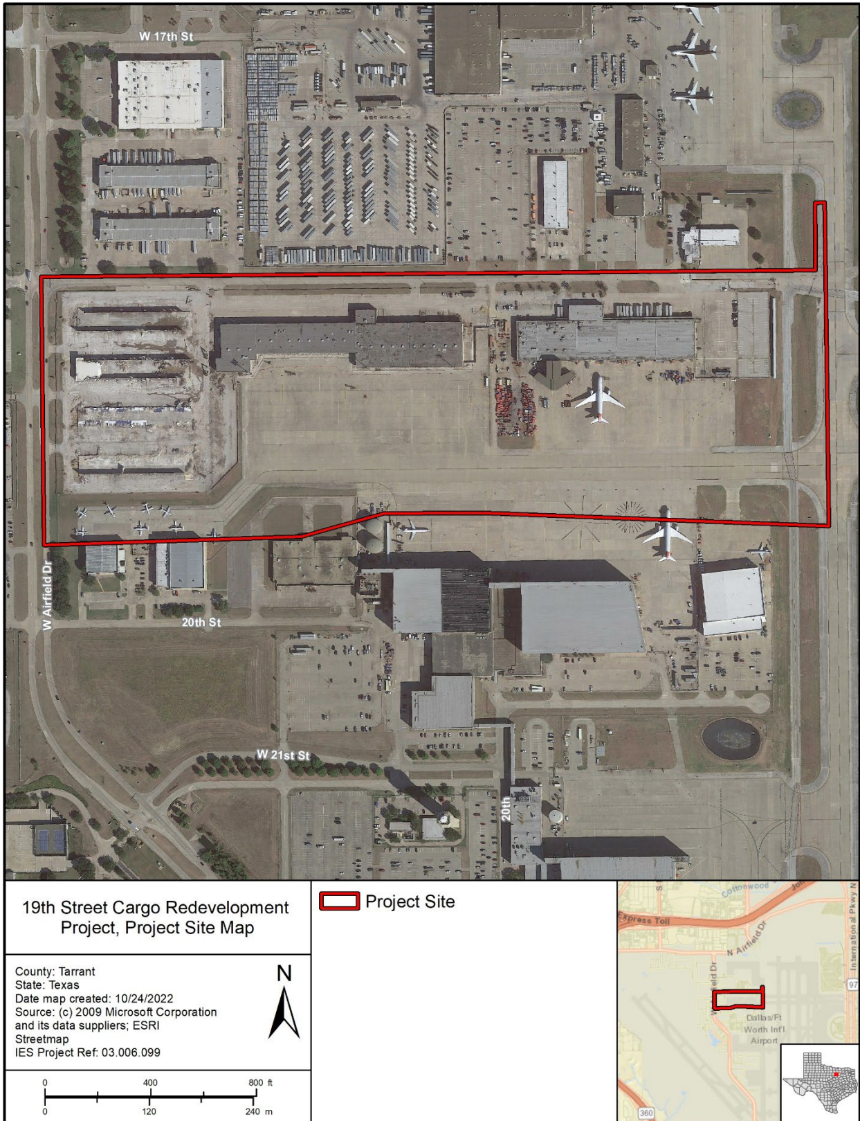
Figure 1. 19 th Street Cargo Redevelopment Project Site, west side of DFW.
