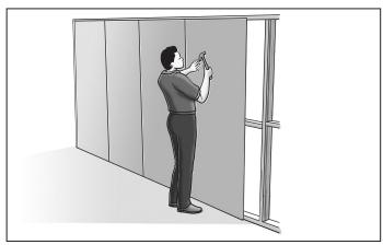
FIGURE 5 SHEET INSTALLATION
