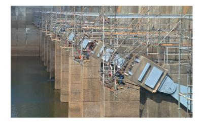
Consequently, the Army Corps had been utilizing a nondestructive testing method at the West Point and Robert F. Henry dams that initiates and records impact vibration response (U.S. Patent 8096195) in the steel tendons without disturbing them. This measured wave motion is compared to the theoretical one and then used to determine the current tension force of the bar tendons in the structures, but the accuracy of this method is limited.
