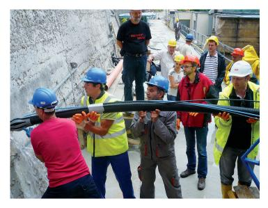
The anchors used were electrically testable El-Iso Strand Anchors in lengths of up to 61.5m. This system has been approved for permanent use (applications with a 100+ year design life).
