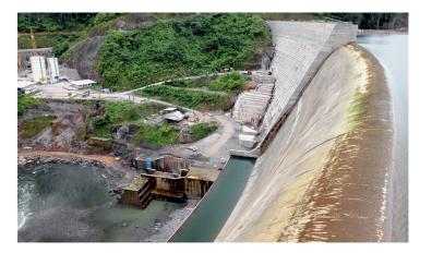
Readings taken during the filling of the reservoir and building pressure on the dam remained within normal limits, which provided a good indication that the anchors had been installed correctly. The combination of the DYNA Force® Sensor readings and anchor restressability provides the capacity to adjust the load at any time during the life of the structure.
