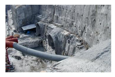
Construction of the Middle Marsyangdi Hydroelectric Power Plant located about 170 km west of Kathmandu, began in 2001. Following completion, the power plant that takes advantage of the natural height of fall of the Marsyangdi river of about 108 m on a 5.5 km long section will generate 72 MW or 400 GWh.
