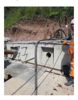
Situated on the Scottish side of the River Tweed, the world's oldest, free-standing, Masonry Pylon road bridge has been restored using the locally sourced Swinton sandstone, quarried by Hutton Stone. The Tower is anchoredto the ground via Compression Struts which, in turn, are bolted to our DYWIDAG PT arrangement cast within the mass concrete ground block. A large fabricated Head Plate were designed and installed to make the final connection through the Thrust Block to the Tension Tie Bars.
