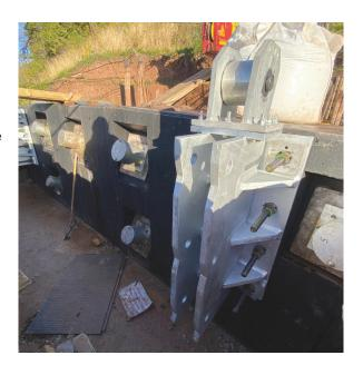
This type of DYWIDAG ground anchor was selected due to the poor or weak ground conditions on the hillside behind the existing stone abutment structure. The Geotechnical engineers (Remedy) were required to design a system of anchoring which would achieve greater anchor loads that were uniformly distributed over the full bond lengths of each 7no Strand Anchors in this location.
