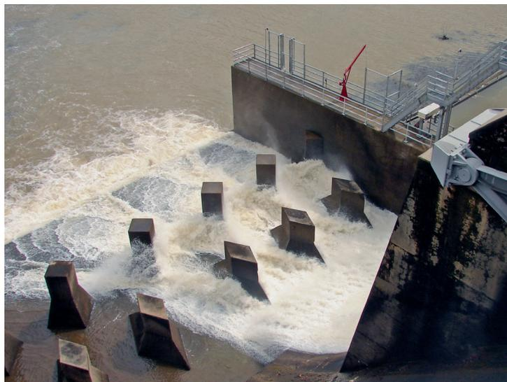
Since 1985, the dam has been regularly tested for seepage, pressures acting on the foundation and deformation. From 2006 to 2008, a two-phased investigative program was carried out that included piezometric measurements, load measurements and core hole drilling through the dam into the foundation.
