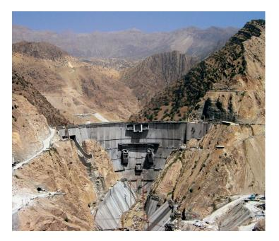
The dam has a length of 388 m with an average thickness of 5.5 m; the total height is 191 m and the foundation width is 29 m. The construction costs for the dam have been assessed at \$150 million. After completion it will be part of an agricultural irrigation system in the South West of Iran.
