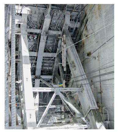
To anchor the trunnion beams of the radial gates to the piers, DYWIDAG supplied a total of 32 27-0.62" DYWIDAG Strand Tendons. The radial gates are located in the center of the dam about 50 m below the crest, and serve to regulate the water level of the dam in case of emergency discharges such as in floods. In addition, DYWIDAG assisted the client by supervising the installation as well as the stressing and grouting of the DYWIDAG Strand Tendons.
