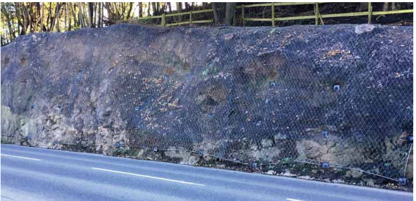
GEWI® Rock Bolts & DELTAX® – Installation at Government House, Jersey
