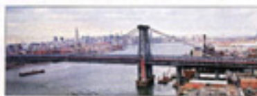
The Williamsburg Bridge once led to a building boom that's now gone down with and quickly followed.
