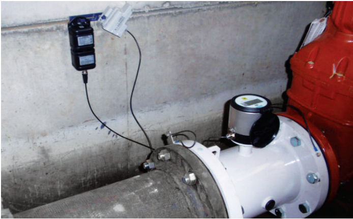
The MAG 8000 is flexible enough for installation virtually anywhere, including district water lines.
