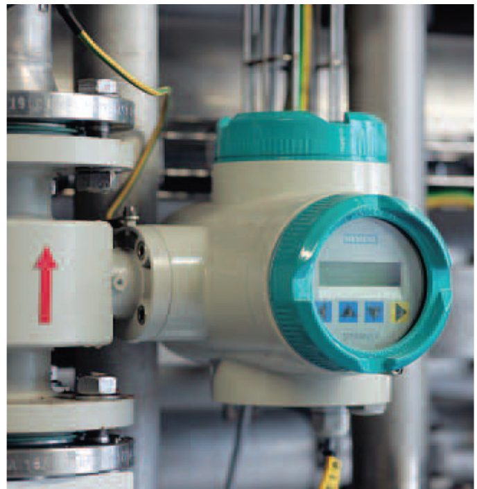
Fig. 4: MAG 3100 Sensor / 6000I Transmitter
