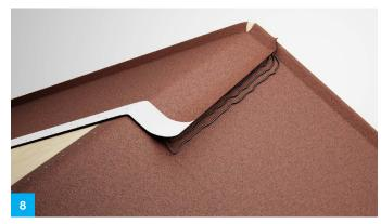
On the opposite side of the roof, lay 150 mm of material over the ridge. Apply glue generously. Press well, so you can see the glue escape at the side. Make a split where the ridge meets the batten. Cover the split at the batten with a piece of TopSafe. Cut the material so that there are no visible nails in the finished roofing.
