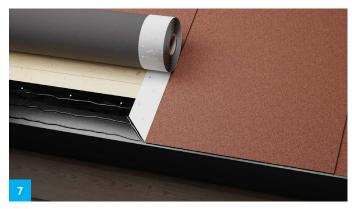
Apply glue to the eave fitting and tread down. Bevel cut to leave as neat a finish as with the previous roll. Apply plenty of glue at the cut.
