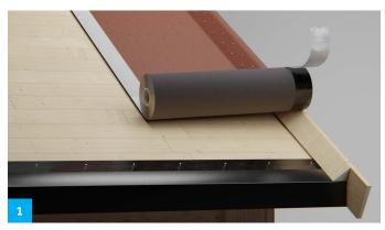
Put TopSafe about 15 cm over the ridge on the opposite side. Align the roll and fasten with roofing nails so that the roll does not twist, see fig. 3. The adhesive edge on the underside must be over the triangular batten. Adjust the length so that a couple of centimetres extends past the eaves. Fit the roll along the triangular batten and rake.
