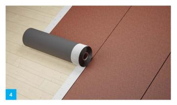
Roll out the next roll, straight over the tear-off strip of the previous roll. Adjust and staple over the ridge.
