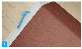
The tear-off strip is perforated in a 60 mm zig-zag pattern. Use galvanized 2.8/25 roofing nails on the perforations. Adjust and staple over the ridge, stretching the material. Start stapling the material from top to bottom. If you have ventilation on your roof ridge, see fig. 14.
