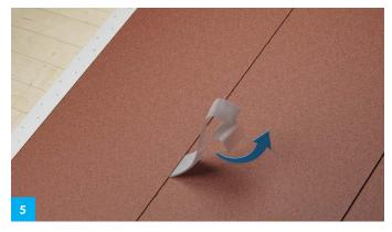
Pull off both strips from the middle going upwards, step on the join, and then pull the strips off down towards the eaves.
