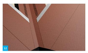
Fit a roll of TopSafe to the valley. Staple the outer edges of the material on both sides. Mark the valley width 200 mm on each side and apply 3 lines of Icopal Roof Glue. Apply strips of TopSafe from each side down into the valley. The glue should leak out as a seal.
