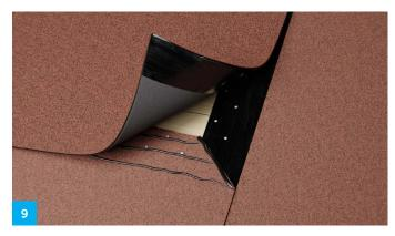
Leave an end overlap of at least 150 mm. Staple in a zig-zag pattern, cut and apply glue generously to the end overlap and the bevel cut. Tread down the overlying part – do NOT nail it. The glue should leak out as a seal.
