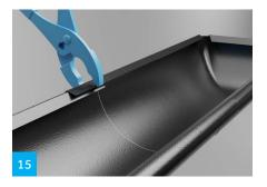
When joining gutters, the folded edge at the back should be squeezed together, e.g. with pliers. Overlap for gutter 4-5 cm.
