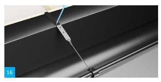
Stay straps should be fitted after the bracket has been mounted. The stay strap is threaded into the hole on the gutter hook and then fastened in the roof batten and down into the counter-batten. In areas with a lot of snow, stay straps/gutter supports must be attached to the rafter with screws.
