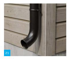
To discharge water into the ground, an elbow is fitted to the downpipe.
