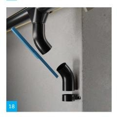
Fit a bend to the downpipe spout. Cut the middle piece from a downpipe 12 cm longer than the distance between the bends.
