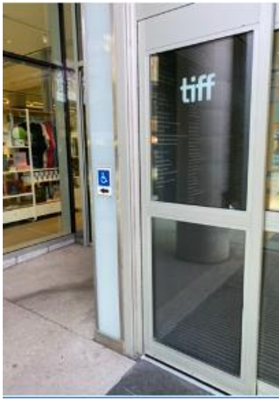
Figure 2: The door on the left side has a pressure sensitive plate for opening.
