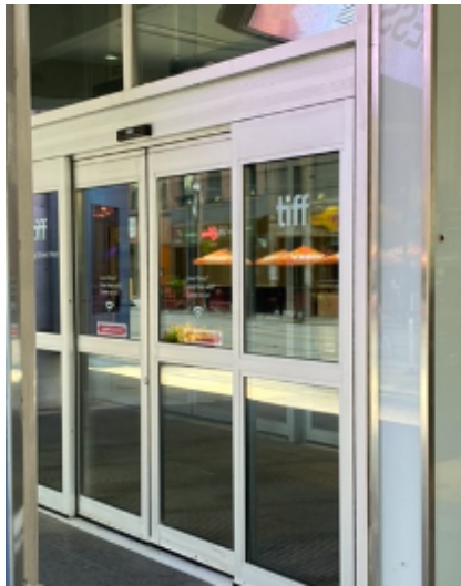
Figure 3: The larger doors on the right side have movement sensors which will automatically open for you.
