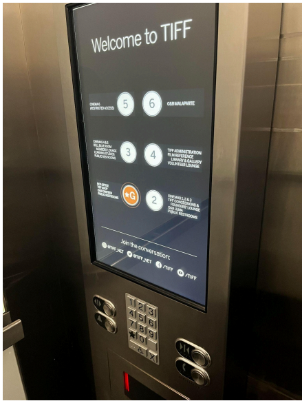
Figure 7: Photograph of elevator touch screen and keypad underneath
