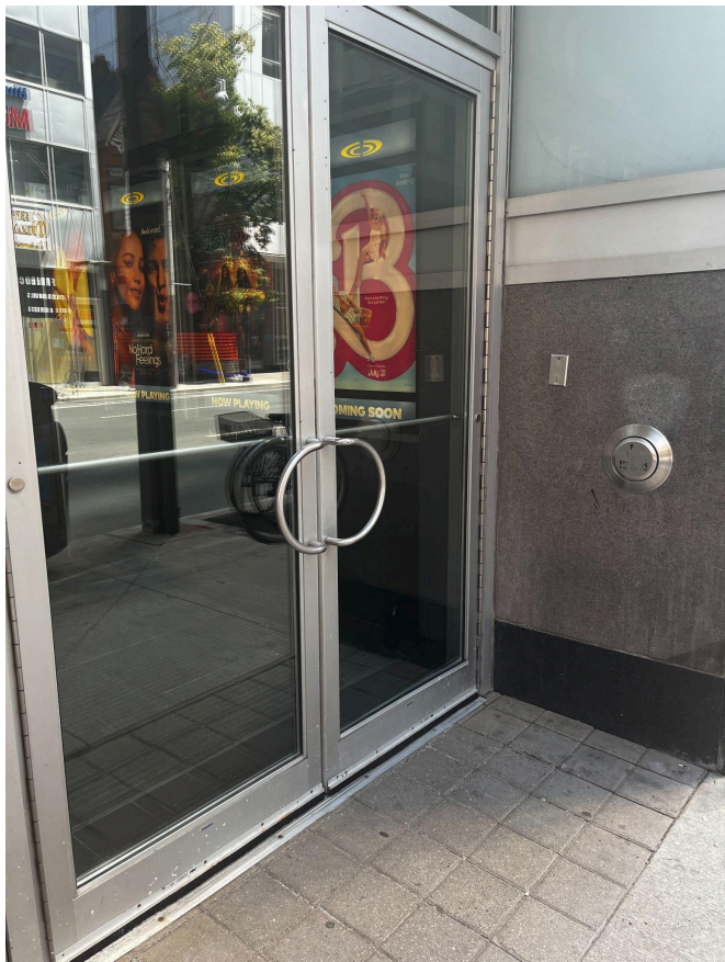
Figure 2: A photograph of the Scotiabank Theatre entrance with the accessible push-to-open button to the right side
