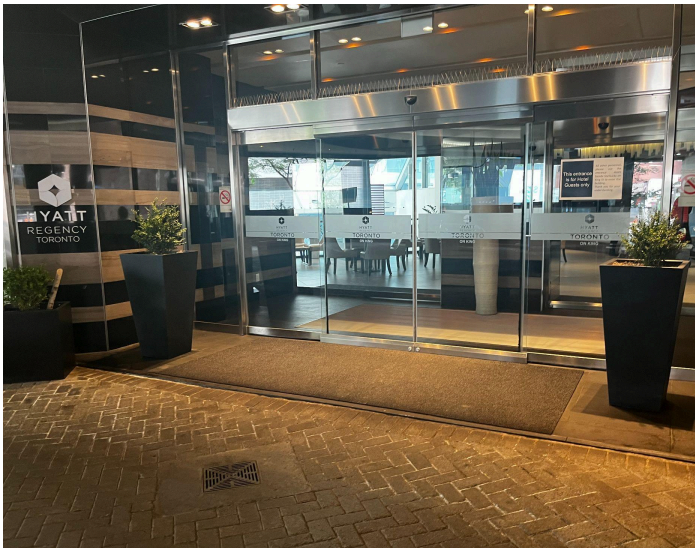
Figure 4: A photograph of the sliding door on Widmer St.
