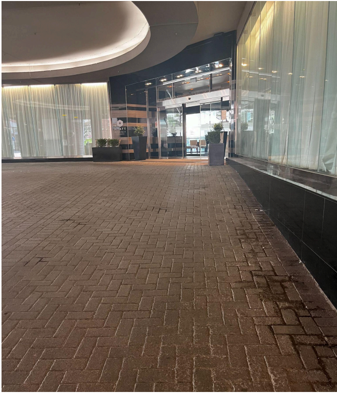
Figure 3: A photograph of the entrance ramp along Widmer St.
