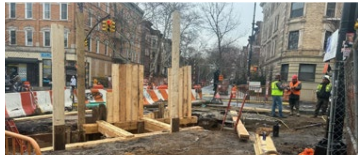
(From top left clockwise) Photos 1 and 2: Storage area on Vanderbilt Ave.; Photo 3: Pest control; Photo 4: Excavation for New 24-inch Reinforced Concrete Pipe on Vanderbilt Ave.
