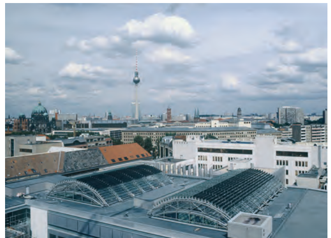
Photovoltaic shading system on the Federal Ministry of Justice, Berlin (Photo: Colt International GmbH, Kleve)
