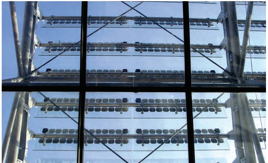
Movable glass louvres with monocrystalline solar cells (Photo: Astrid Schneider)
