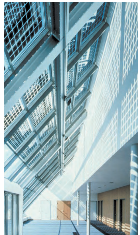
Federal Ministry of Economics and Labour: Solar cells integrated into insulated glazing (Source: Scheuten Solar Technology GmbH)
