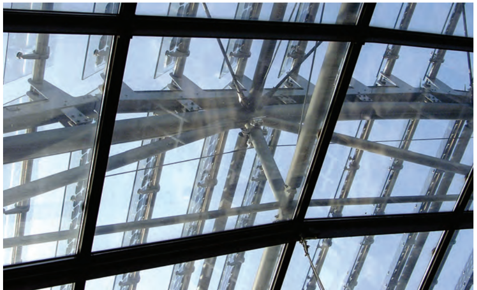
Insulating glazing attached to the underside of the lattice girders with steel cables (Photo: Astrid Schneider)
