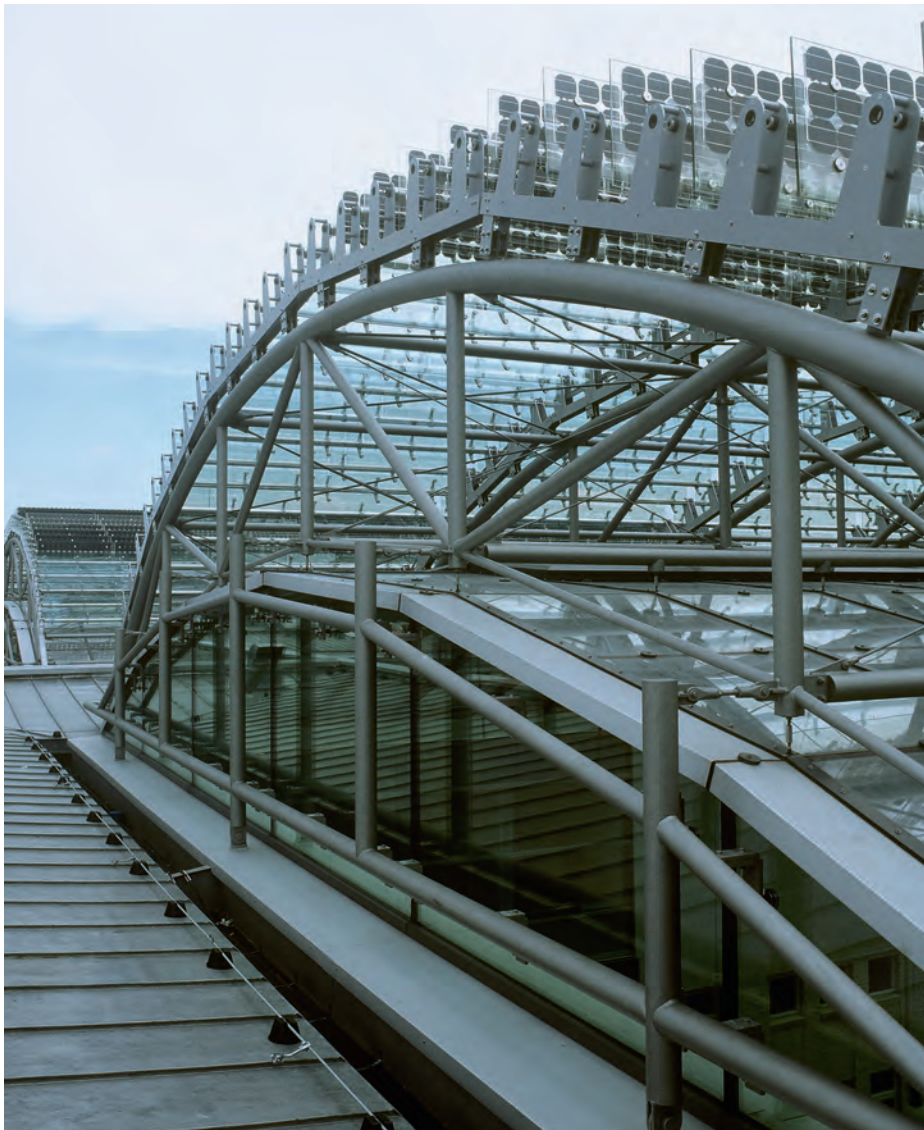
Glass louvre system with solar cells (Source: Colt International GmbH)
