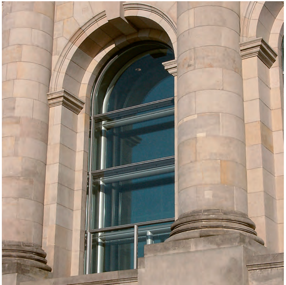
Facade double window: safety glass with open joints to the frame (outside) and insulating glazing (interior) to permit natural ventilation. (Photo: Astrid Schneider)
