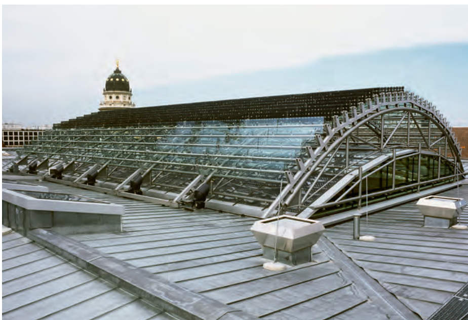
Shading system of glass louvres with and without solar cells (Source: Colt International GmbH)
