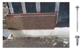
**2.** Start from a corner. Lap orientation is not relevant. Minimum 4 screws per board.
