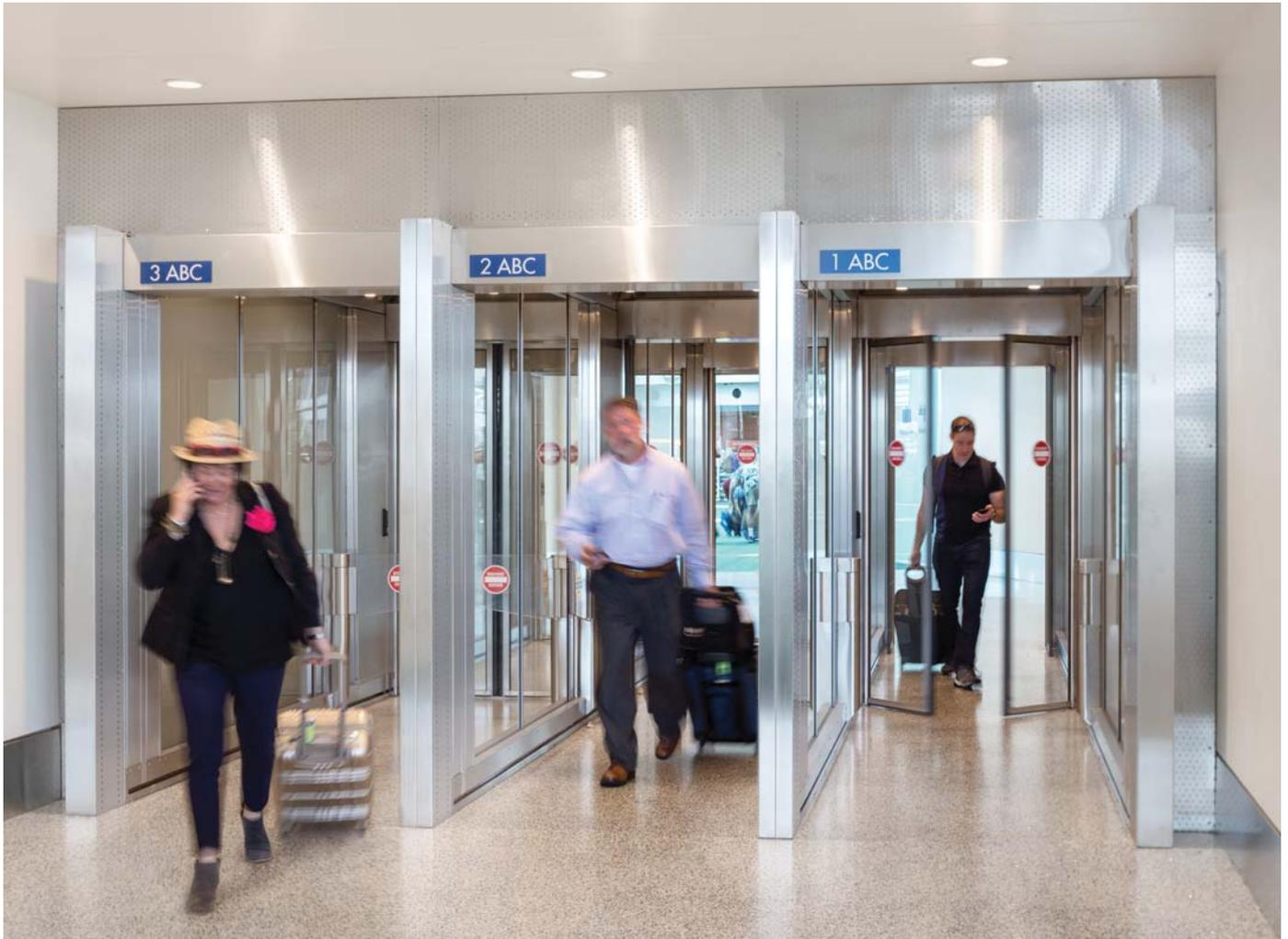
Ensures safe passage in a permitted direction when there is a large number of people. The door detects and inhibits passage attempts in the unauthorized direction.
