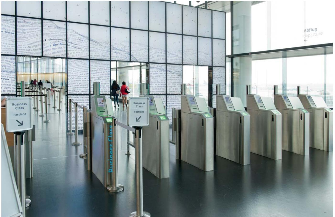
Waist-high sensor barrier, designed as an e-gate in the terminal. Helps staff ensure controlled access to the security area – smoothly and efficiently.
