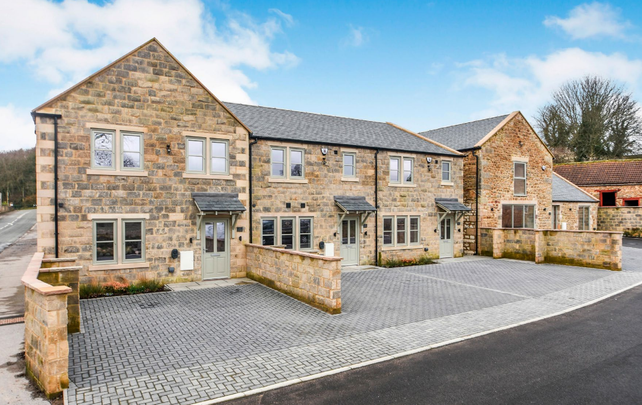
BRAMBLE COTTAGE, CARR COTTAGE AND IVY COTTAGE Village Farm, West Tanfield
