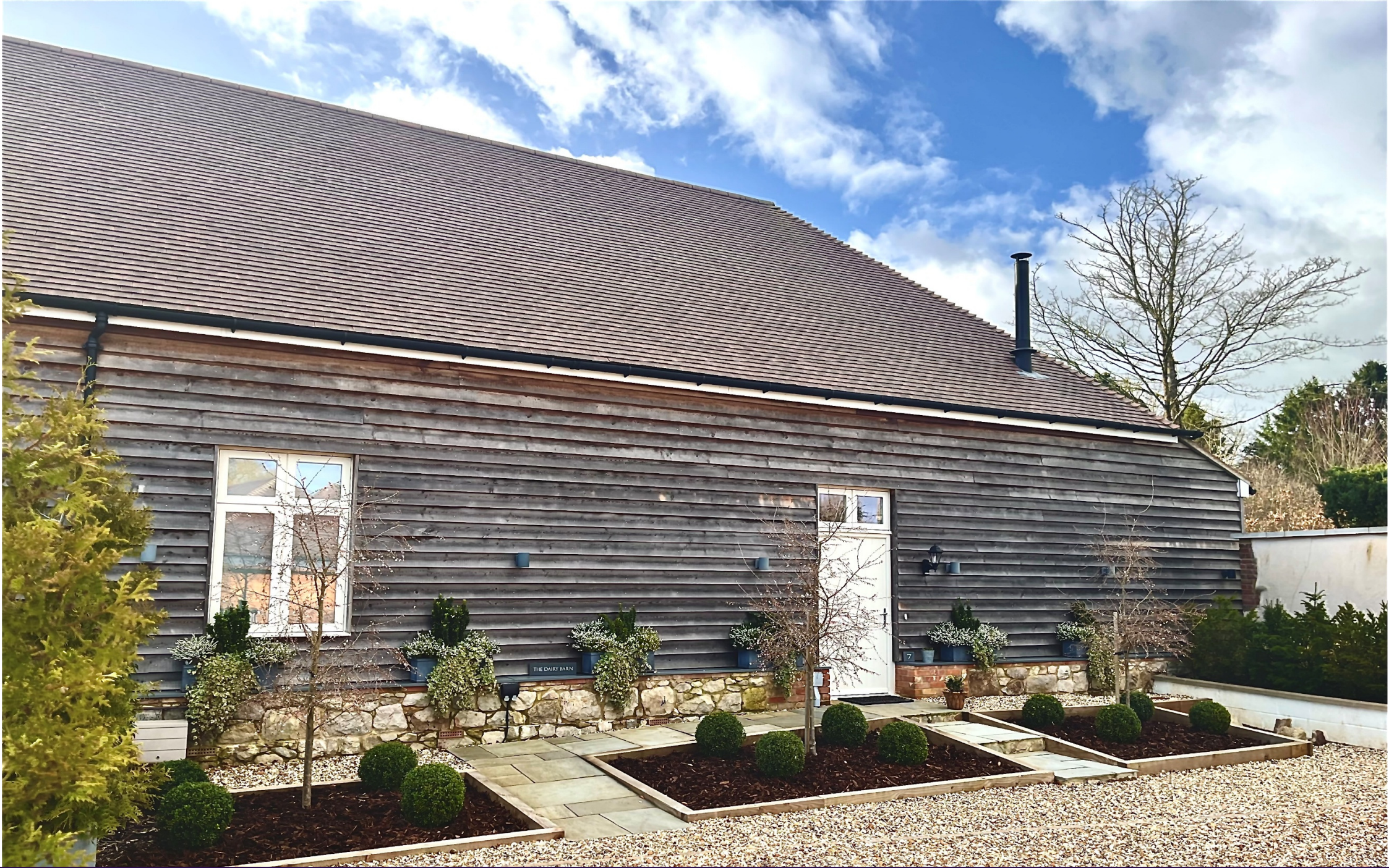
THE DAIRY BARN, OLD DAIRY LANE, WINTERBOURNE MONKTON
