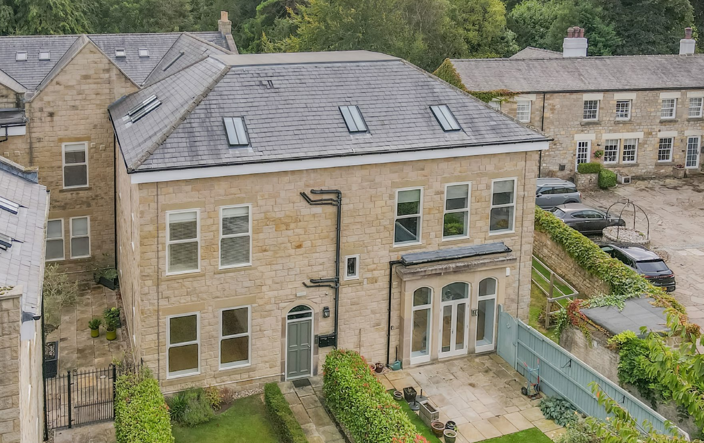
Apartment 14, Linton Springs Wetherby
