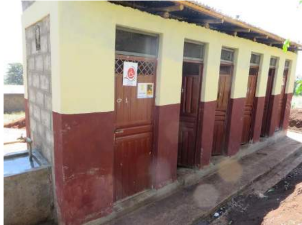
1 PHOTO OF THE SANITATION HARDWARE
