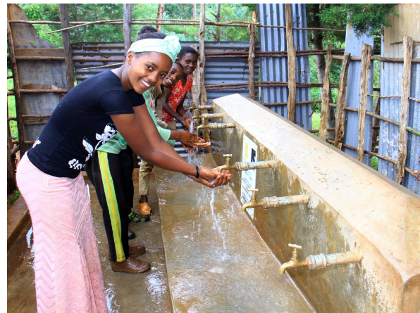
1 PHOTO OF THE HANDWASHING STATIONS
