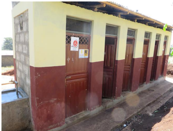
1 PHOTO OF THE SANITATION HARDWARE
