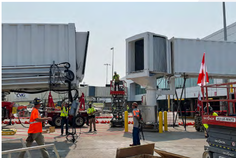
Passenger boarding bridge being installed at Concourse B
