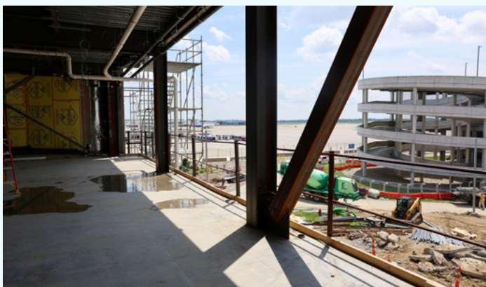
Main terminal East and West enclosure expansion
