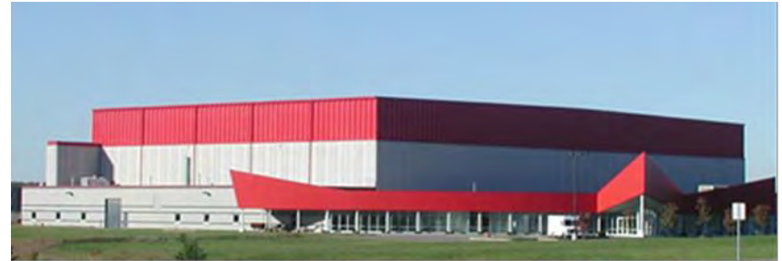
Photo: Pemco Maintenance Hangar, CVG
