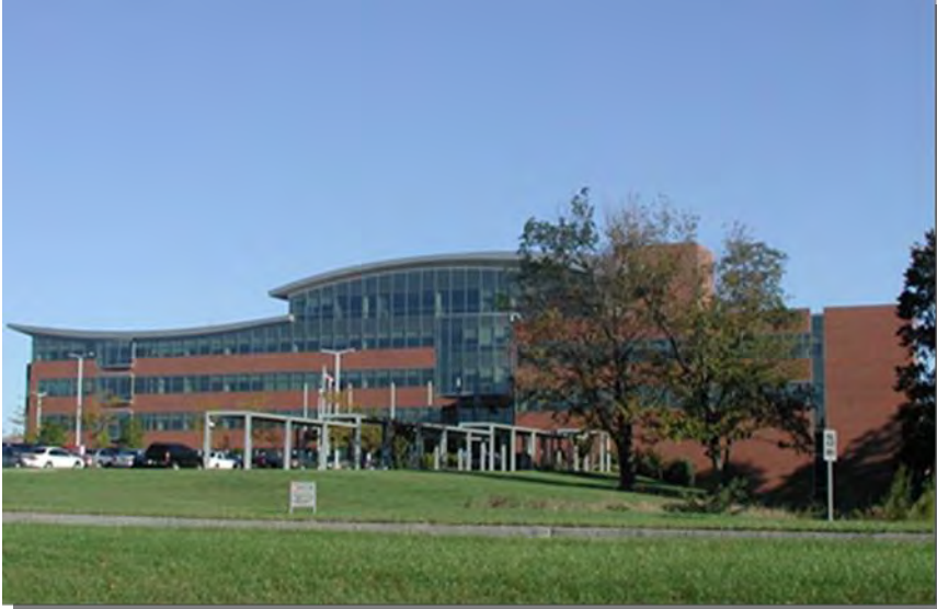
General Office Building, South Airfield
