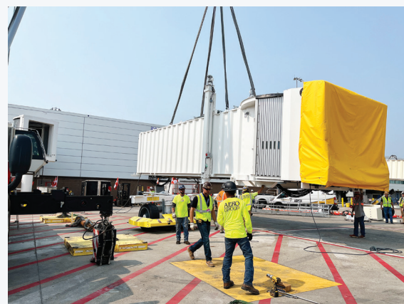
Over the next two and a half years, CVG will install 28 new passenger loading bridges in Concourse B. This is the first one being installed in June.
