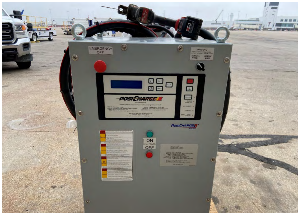
Figure 3. Charging Station for Electric Ground Support Equipment at CVG
