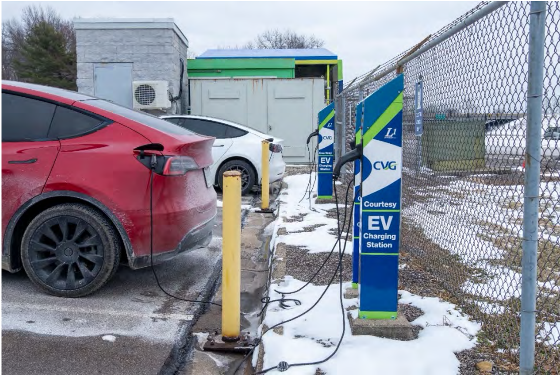
Figure 1. Level 1 Charging Stations at CVG ValuPark Lot
