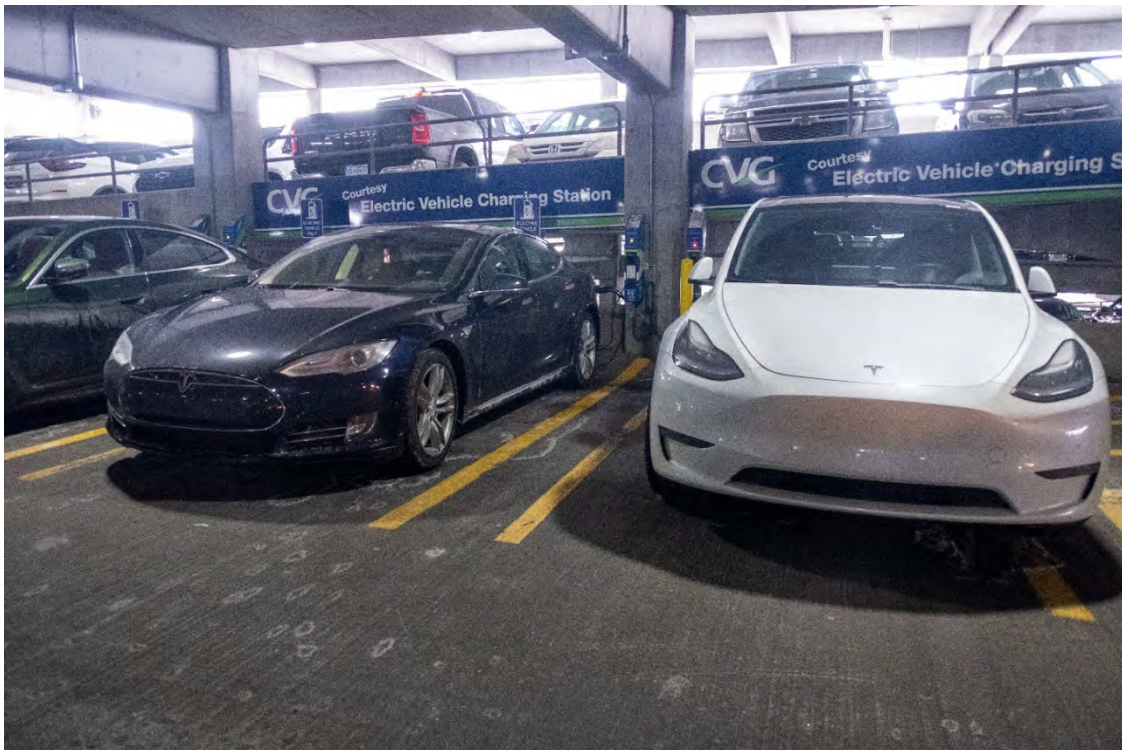
Figure 2. Level 2 Charging Stations in Terminal Parking Garage
