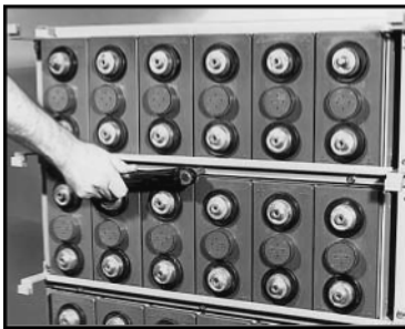
Figure F1. Removal of cell retaining bar
