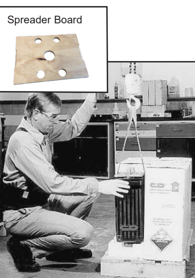
FIGURE 1.4.2 - Use of lifting sling and spreader board
