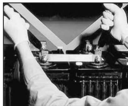
Figure 11.6.1 - Measuring connection resistance with
