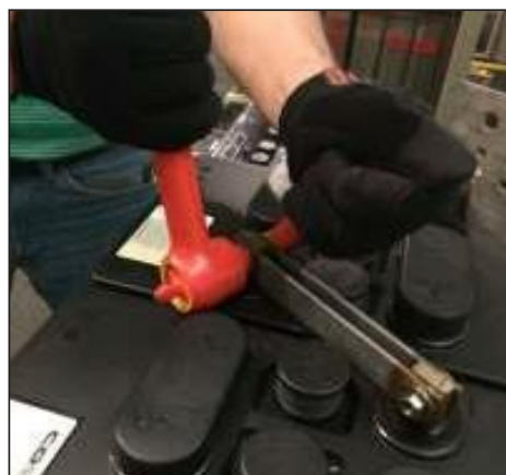
Figure 4.6.3 – Torquing Connections
