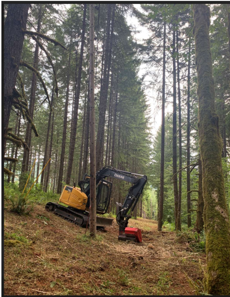
Figure 16: SlashBuster Clearing Right-of-Way
