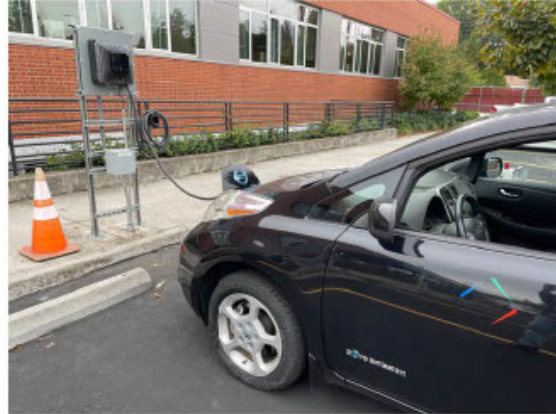
Fig. 1. A Nissan LEAF undergoing V2G testing at PGE's Portland Service Center with a Quasar Wallbox charger. The 240 V, 32 A bi-directional charger can provide up to 7.2 kW of power from the vehicle battery to the grid. Successful testing of the charger's V2G capability was conducted in October 2021, with ongoing efforts underway to study the efficiency and reliability of the charge/discharge process.
