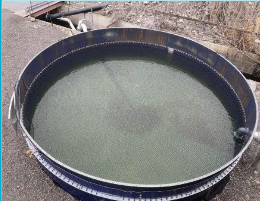
Current temporary stress relief pond
