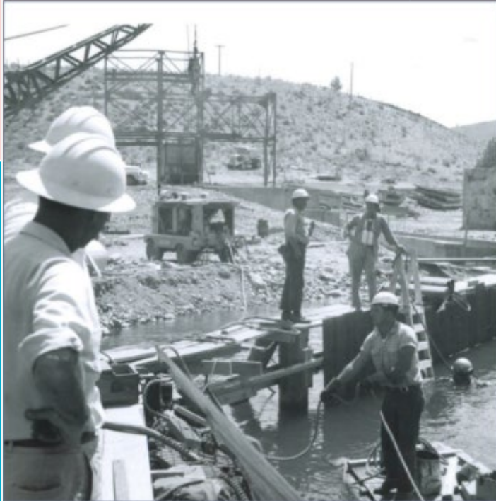
Pelton Trap construction - 1956
