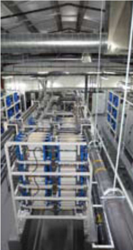
Vanadium Redox Flow Battery (Source: Prudent Energy brochure)
