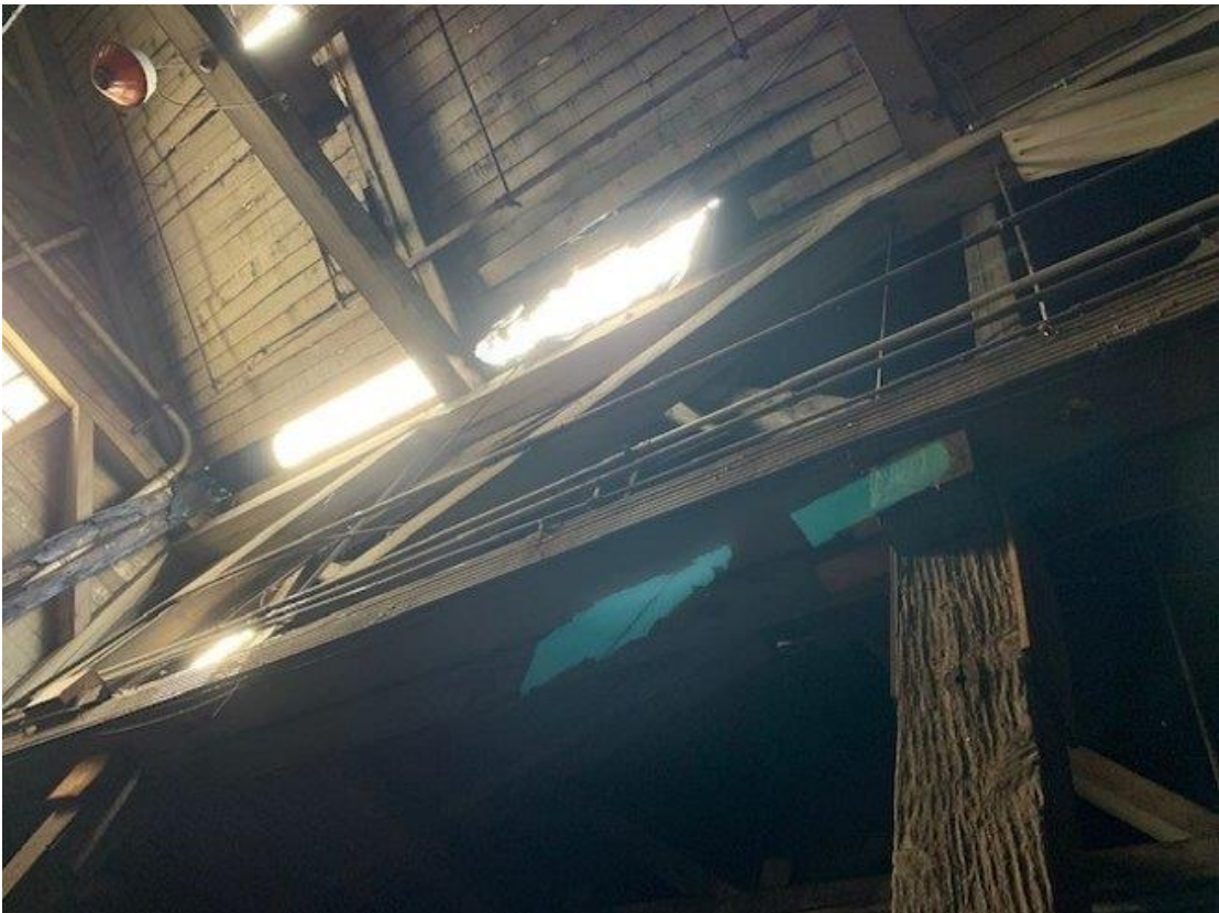
Decayed roofing
