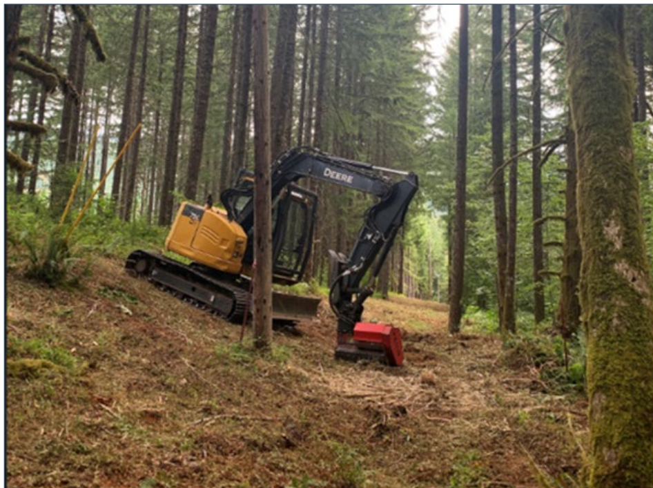
Figure 23. SlashBuster Clearing Right of Way
