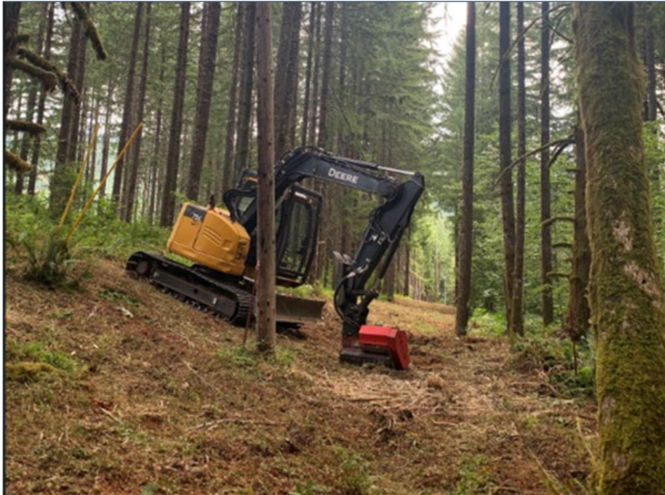
Figure 23. SlashBuster Clearing Right of Way
