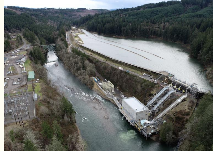
Faraday Hydro Facility
