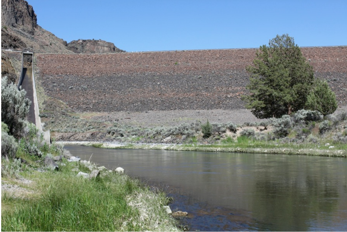
Bowman Dam East dam retaining wall
