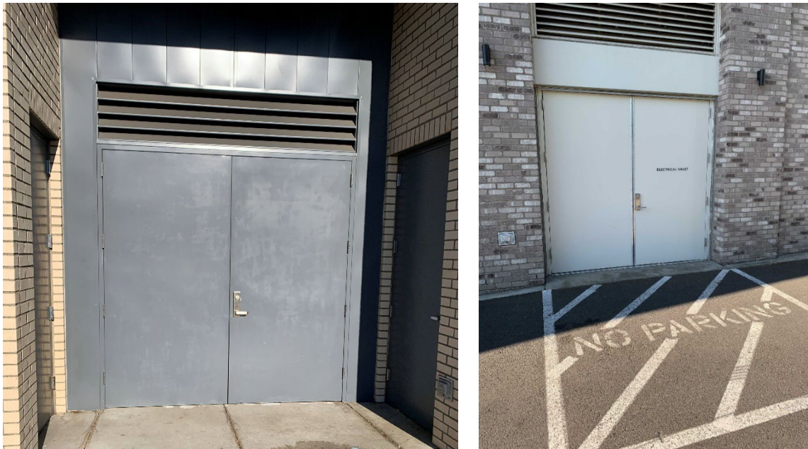
Figure 6. Equipment Access Double Doors for At-Grade Vaults
