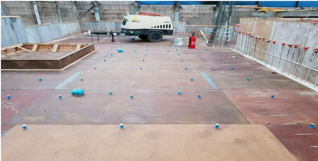
Figure 28. Installed Ceiling Grid
