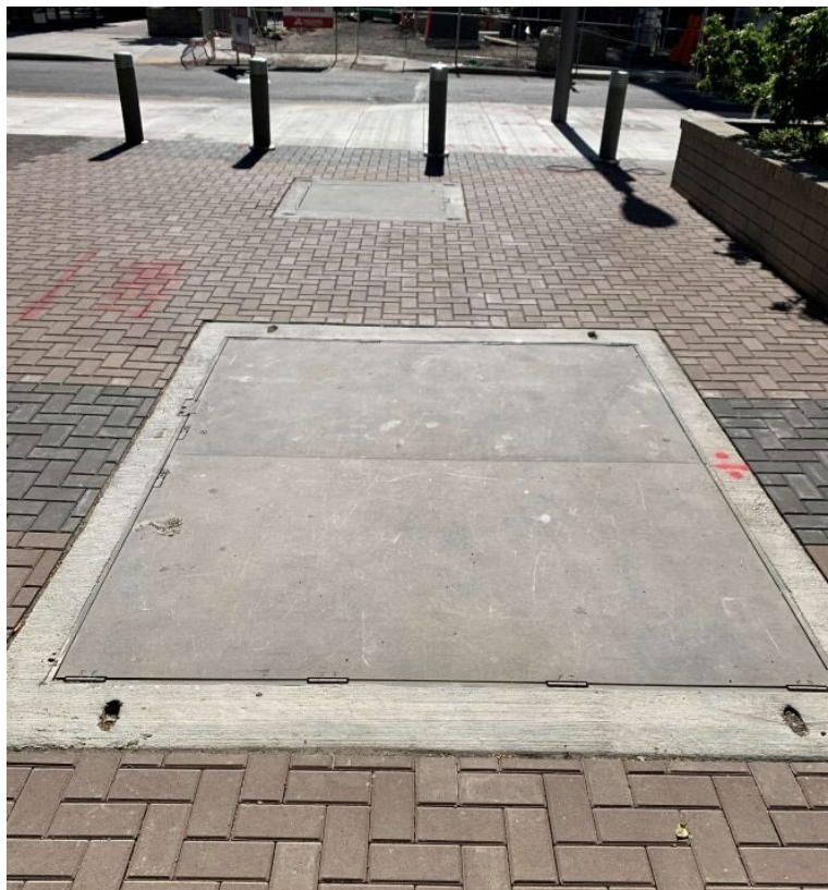
Figure 8. Equipment Access Hatches for Sub-Grade Vaults Foreground: Equipment Access Hatch; Background: Personnel Hatch (a.k.a. Man Door)
