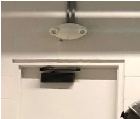
Figure 24. 1100 L “Bug-Eye” Emergency Egress Lights
