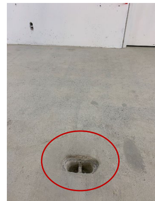
Figure 23. Installed Spread Anchor Receiver
