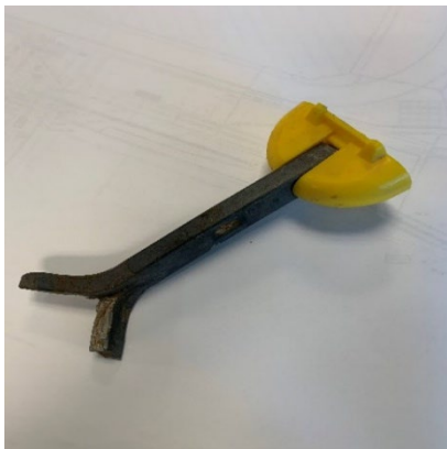
Figure 21. Spread anchor receiver with mounting cup
