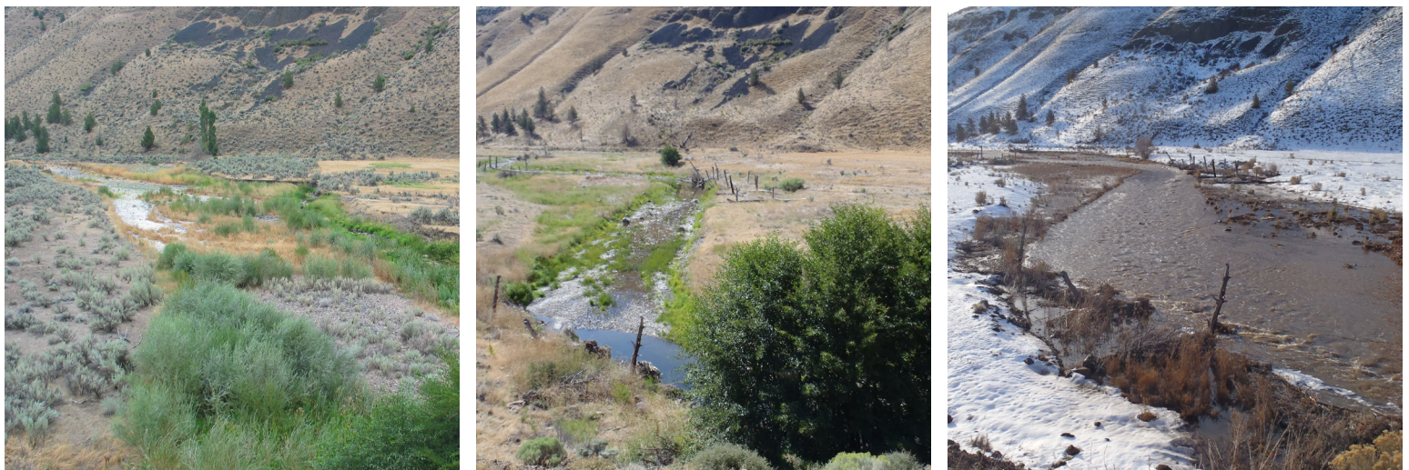
Before restoration (left): the Trout Creek channel banks were incised and easily eroded. After restoration (center and right): the project restored a meandering channel with wide floodplains and opportunities for riparian growth.
