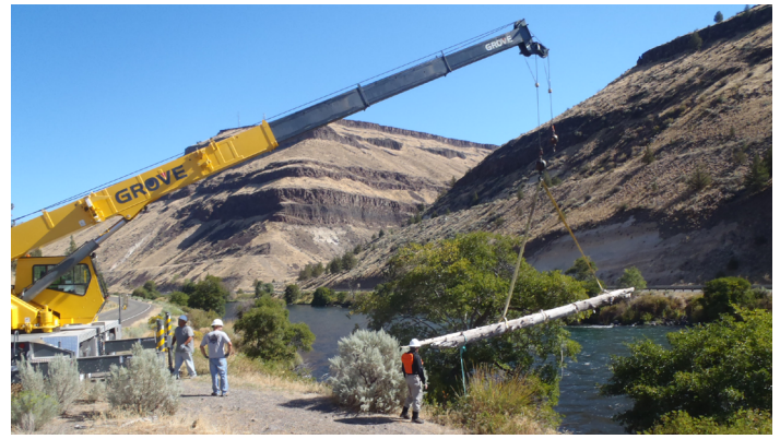
PGE crews use cranes to place logs in locations and configurations that mimic naturally-transported wood.
